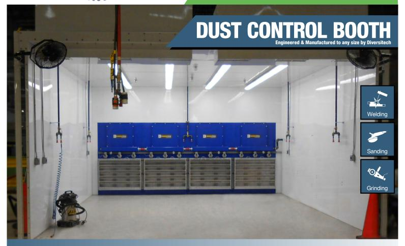
Diversitech's Dust Control Booth are designed to safety capture and filter airbone contaminants from metal finishing, fiberglass, composites and metal fumes.
